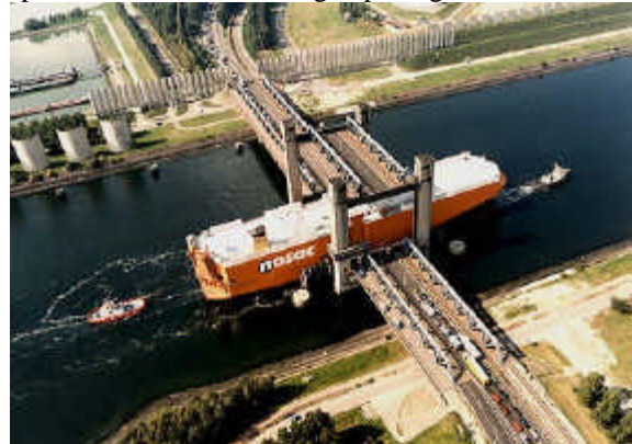
Figure 1: typical tow operation
